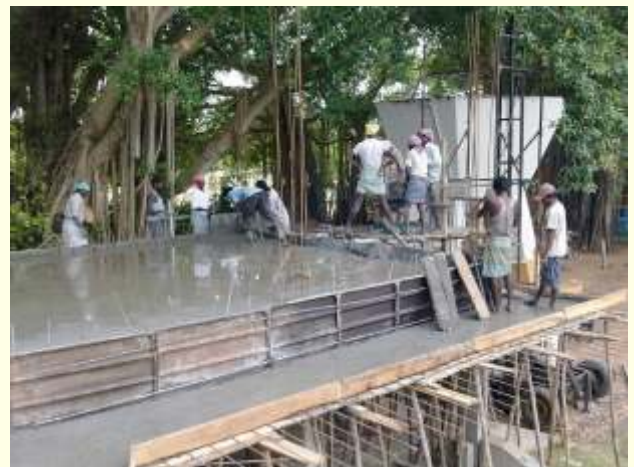
The concrete was poured in 1 day
